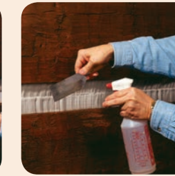
4. Lightly mist the trowel as needed.
