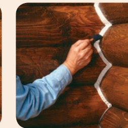
4. Tool to ensure a tight seal to the top and bottom of the chink line.
