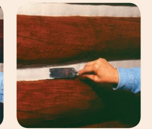
5. Tool to ensure a tight seal to the top and bottom of the chink line.
