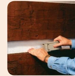
2. Tape the entire joint using polyester tape.
