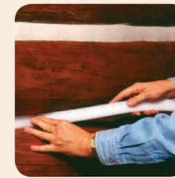
1. Install Grip Strip into caulk well of clean, stained logs.
