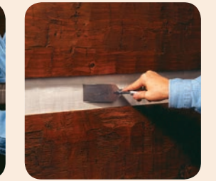
5. Tool to ensure a tight seal to the top and bottom of the chink line.
