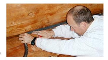
Backer Rod is flexible and compressible; it conforms to the irregularities in the log surface. Its primary function is recognized as a median between the log gap and the chinking. Select the proper Backer Rod that fits flush with the logs.
